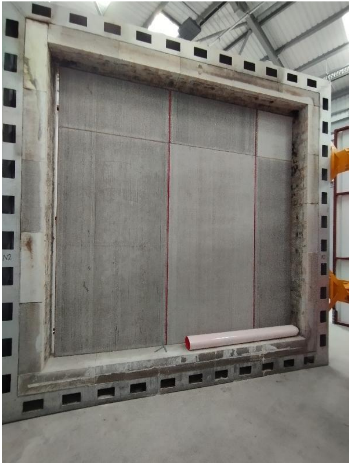
Photograph 7 – Sheathing board layer fitted.
