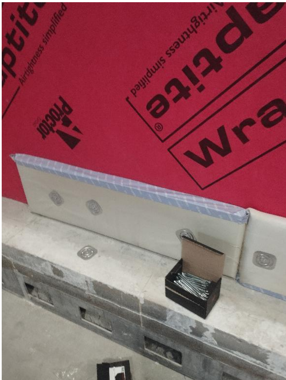
Photograph 9 – Alpha pad being secured
