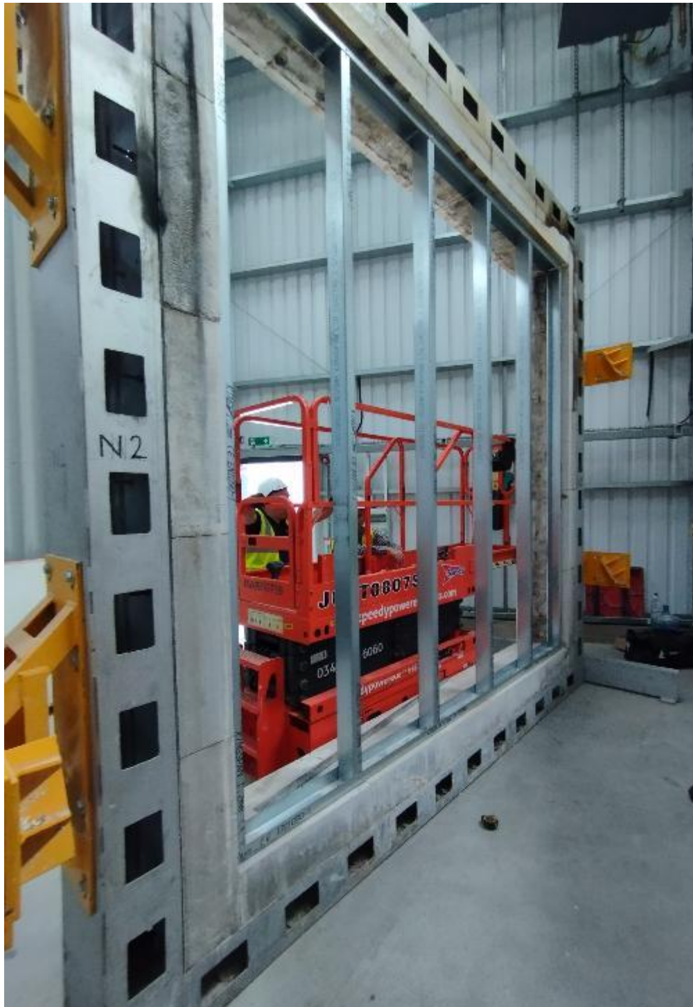
Photograph 1 – Steel frame construction fixed to frame
