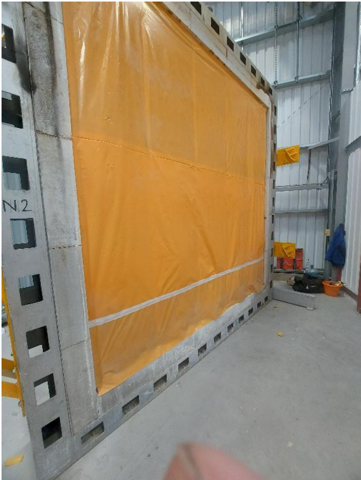
Photograph 4 – Layer of Visqueen applied to fireside
