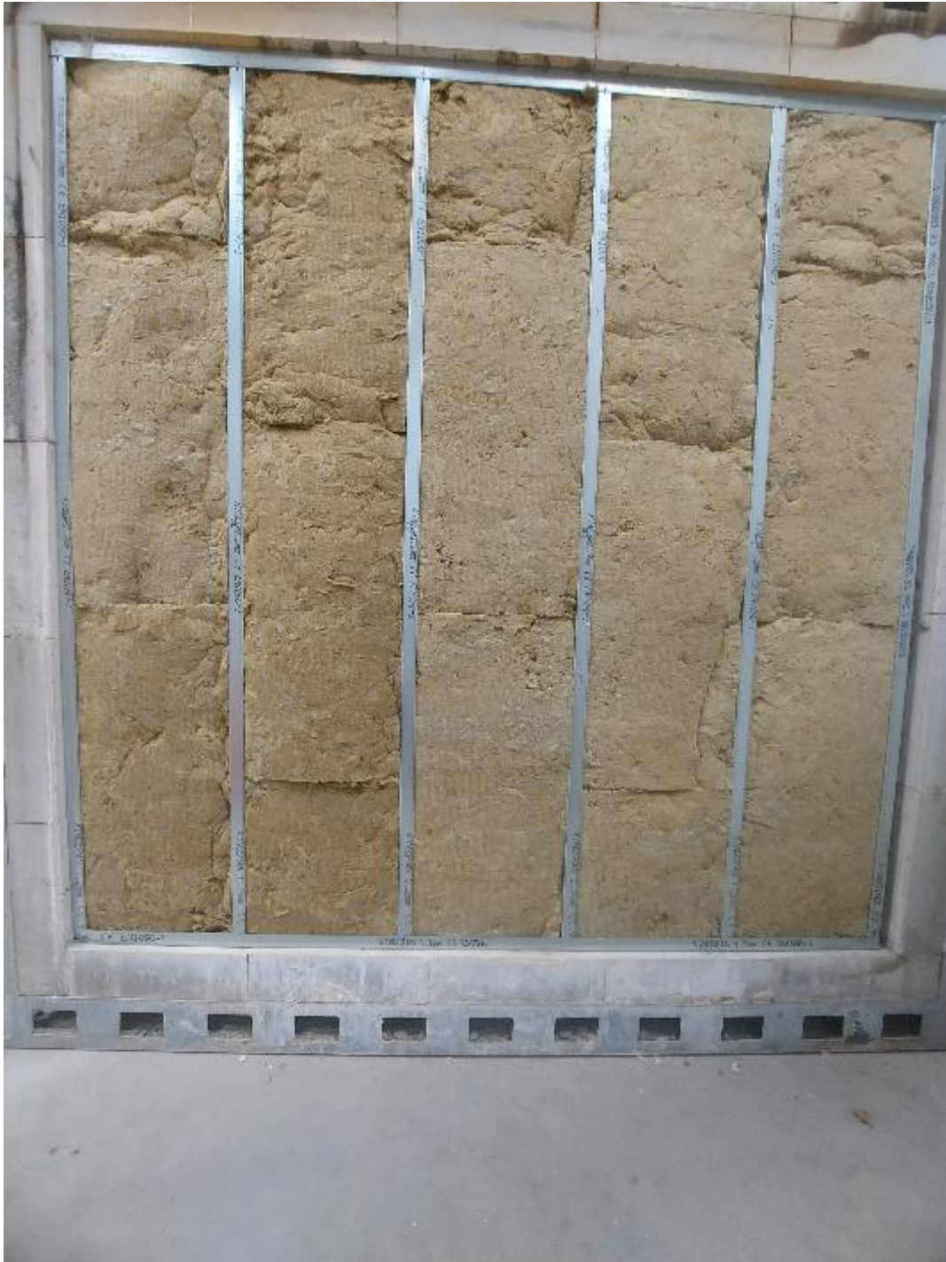
Photograph 3 – Insulation fitted into SFS
