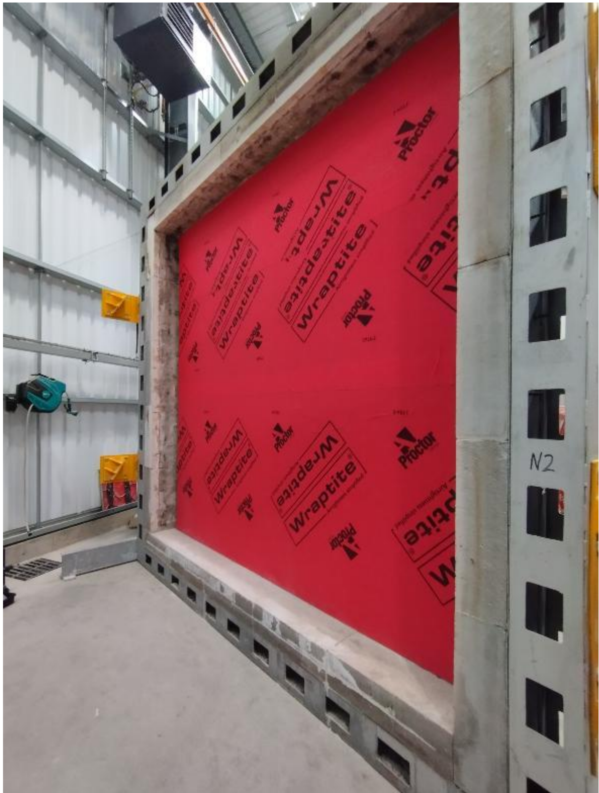
Photograph 8 – Wraptight fitted over sheathing layer.
