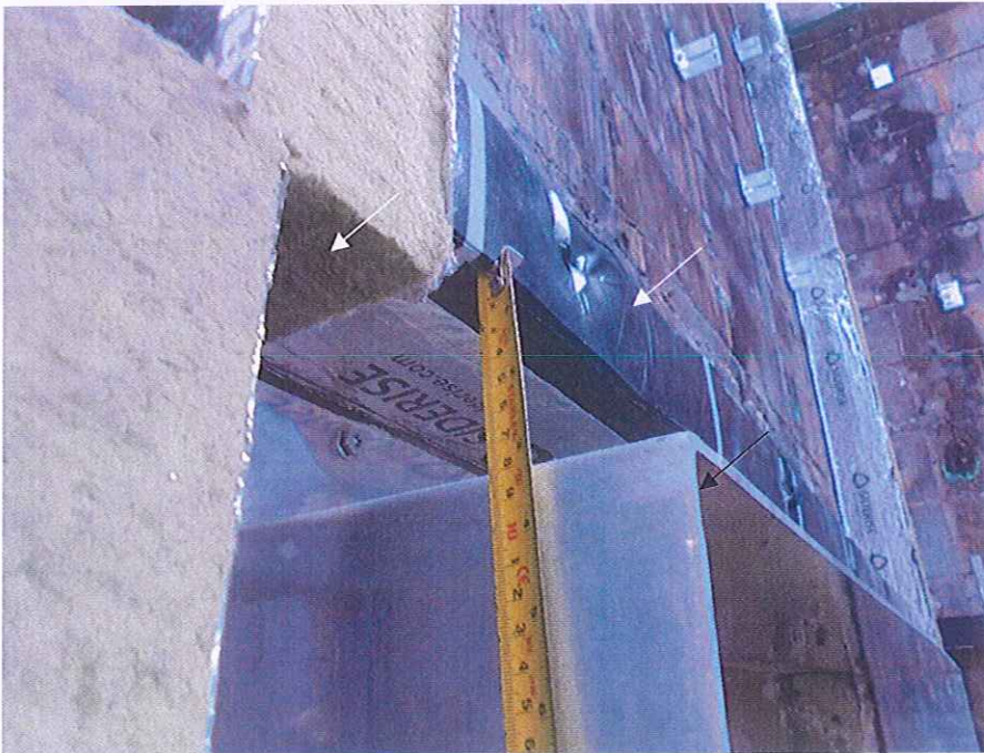
Aluminium flashing and horizontal intumescent cavity barrier above combustion chamber
