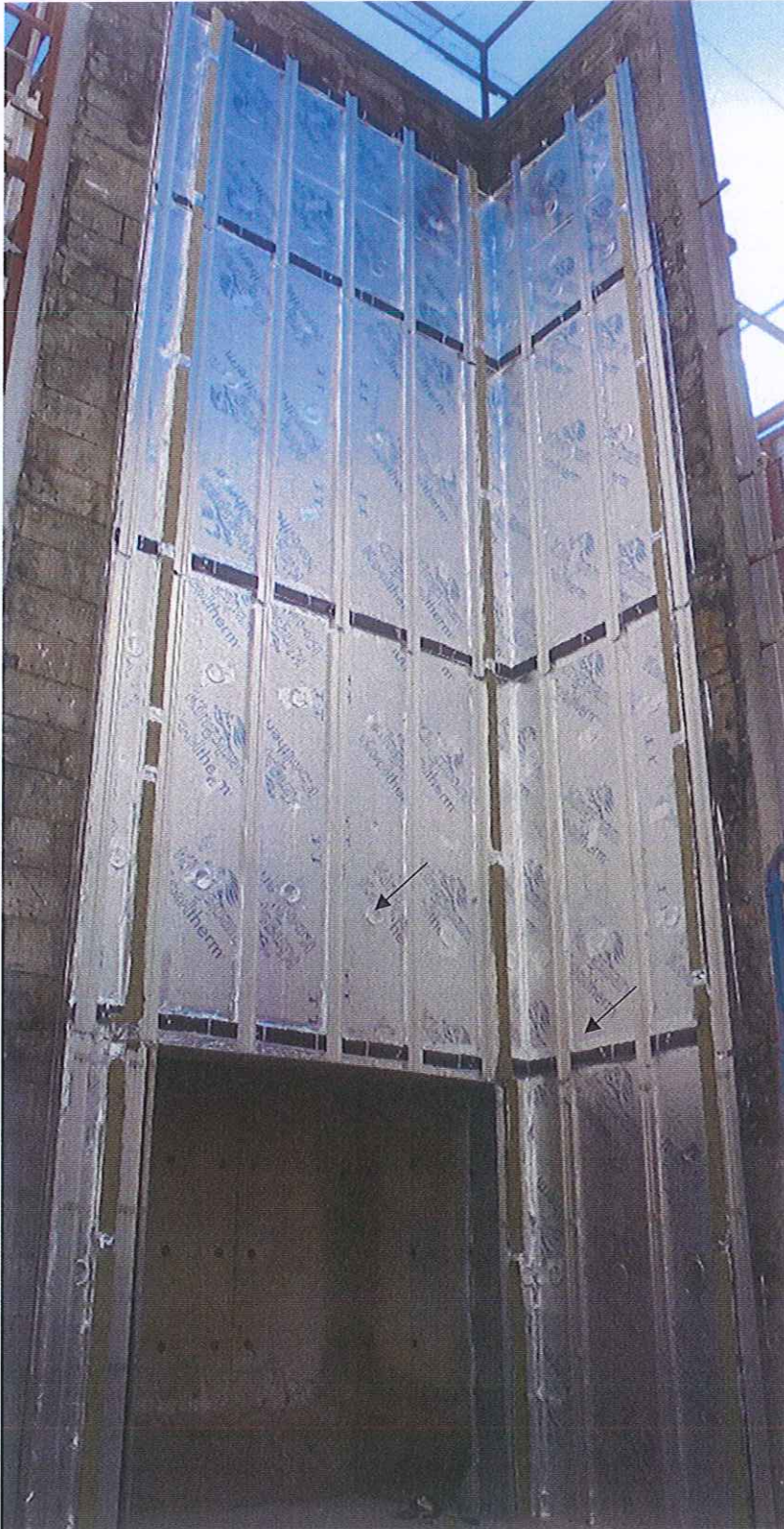
Kooltherm K15 insulation 100mm & aluminium foil tape
