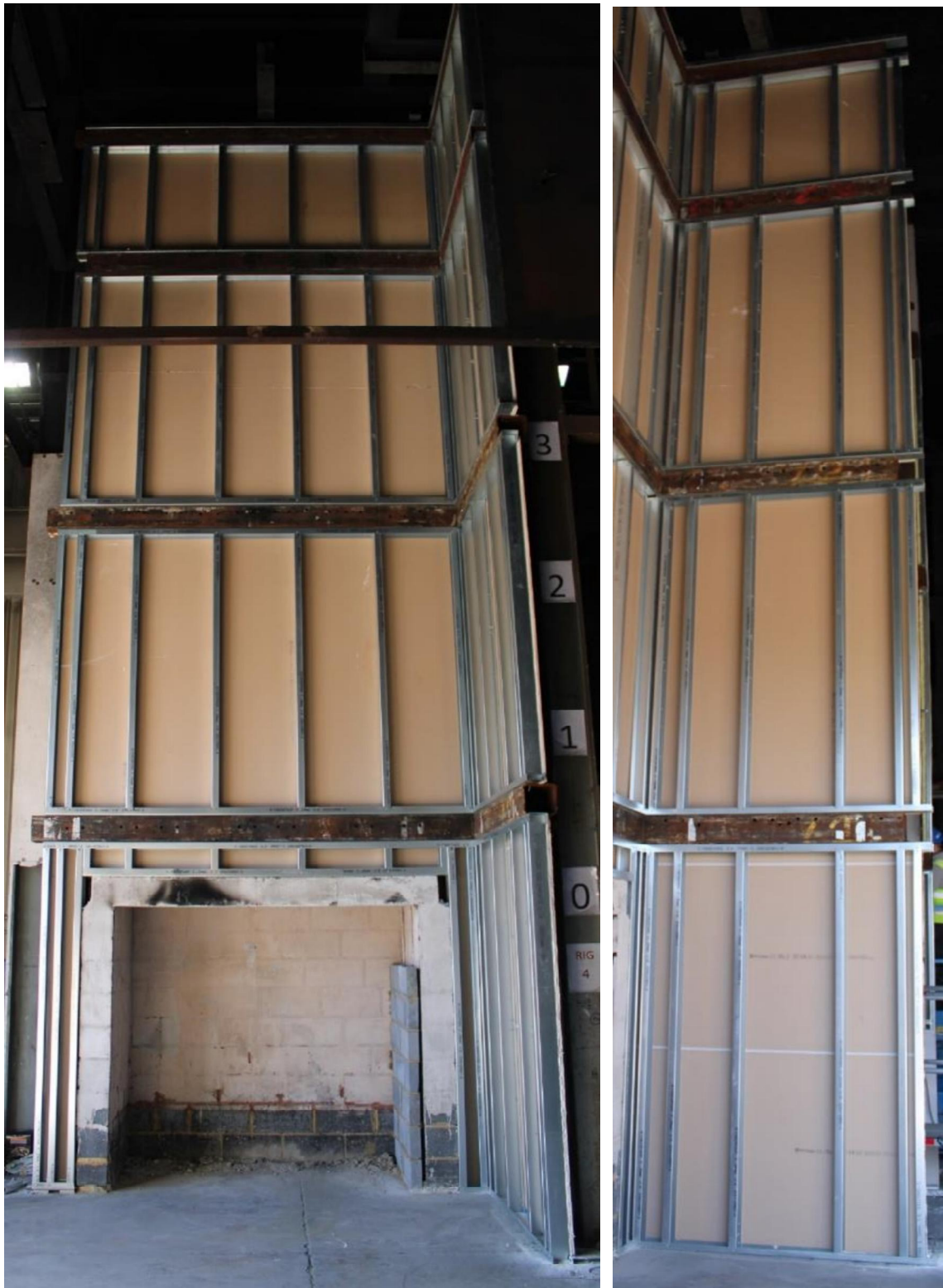
Figure 3. Full-height installation of the steel framing system and plasterboard.
