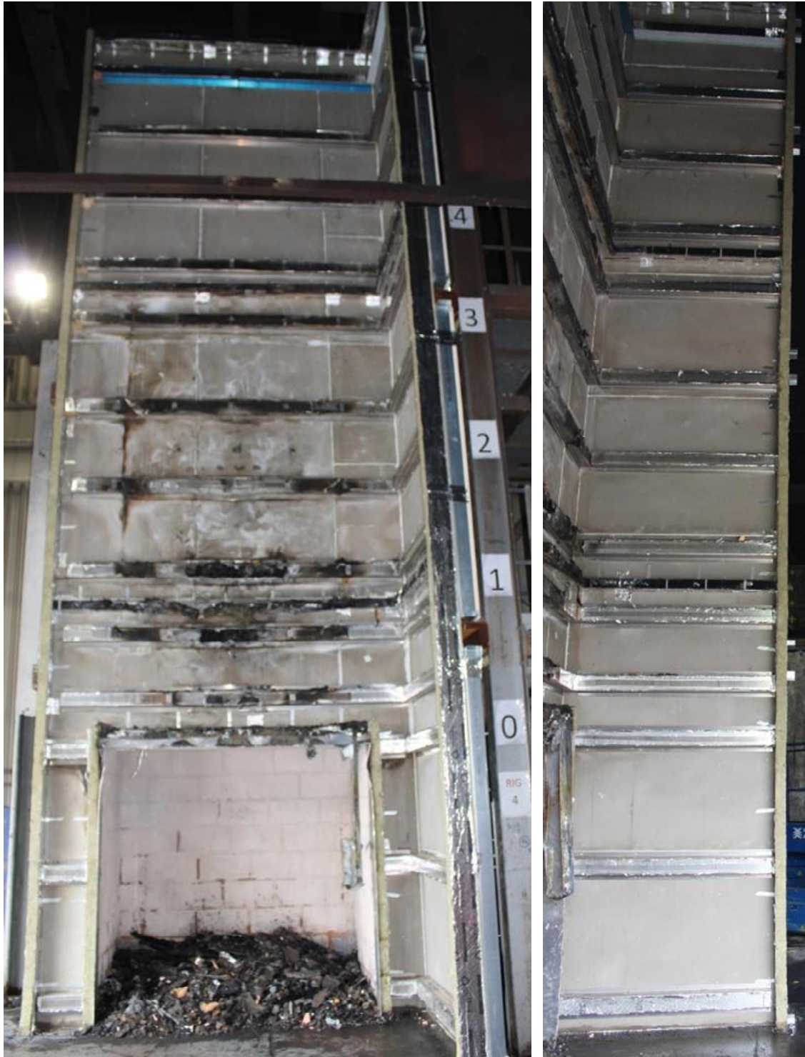
Figure 55. Full-height photograph following removal of insulation and brackets.
