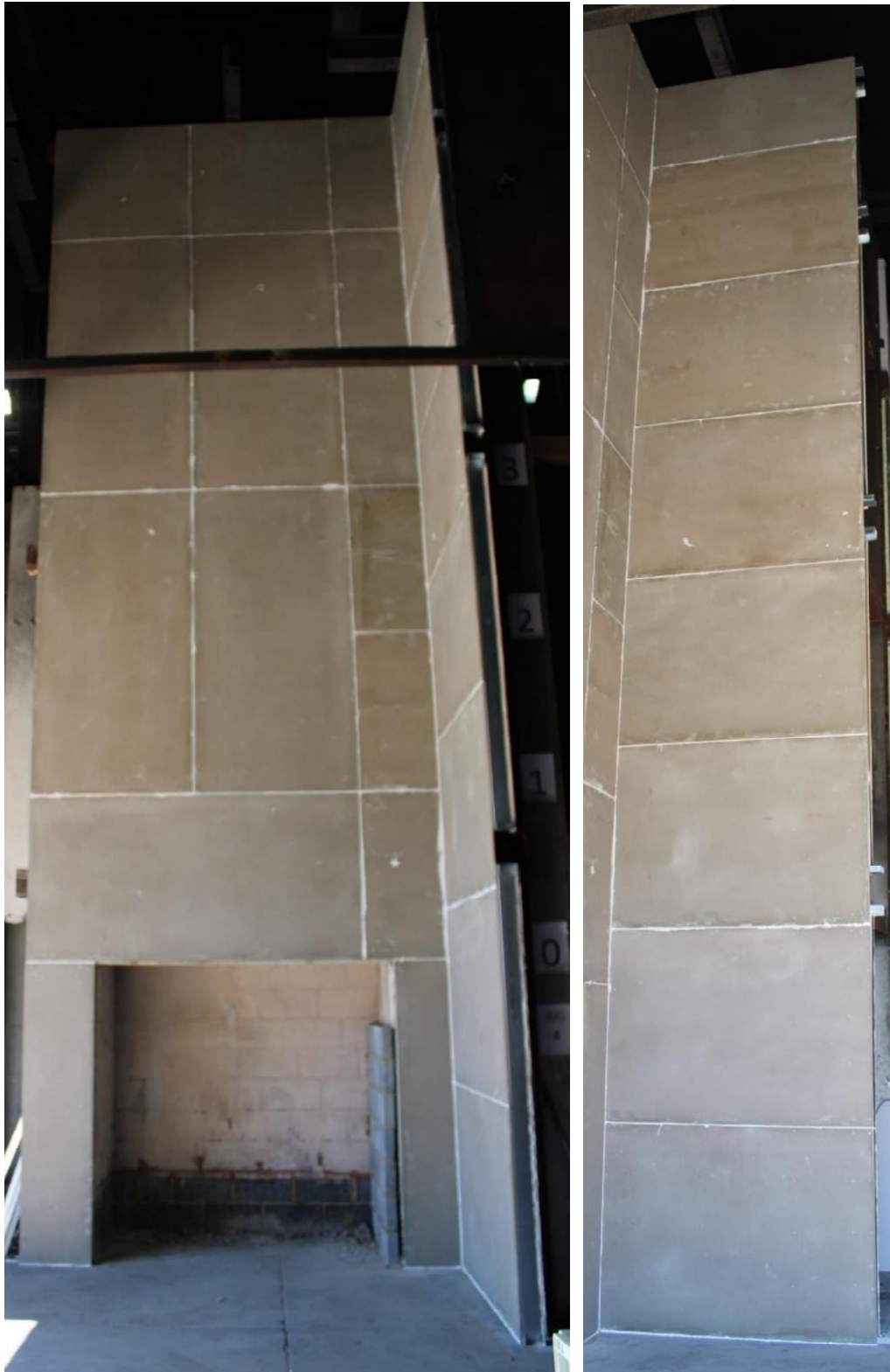
Figure 6. Full-height installation of the sheathing board.
