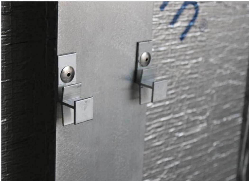
Figure 25. Centre double clip fixed to rail.
