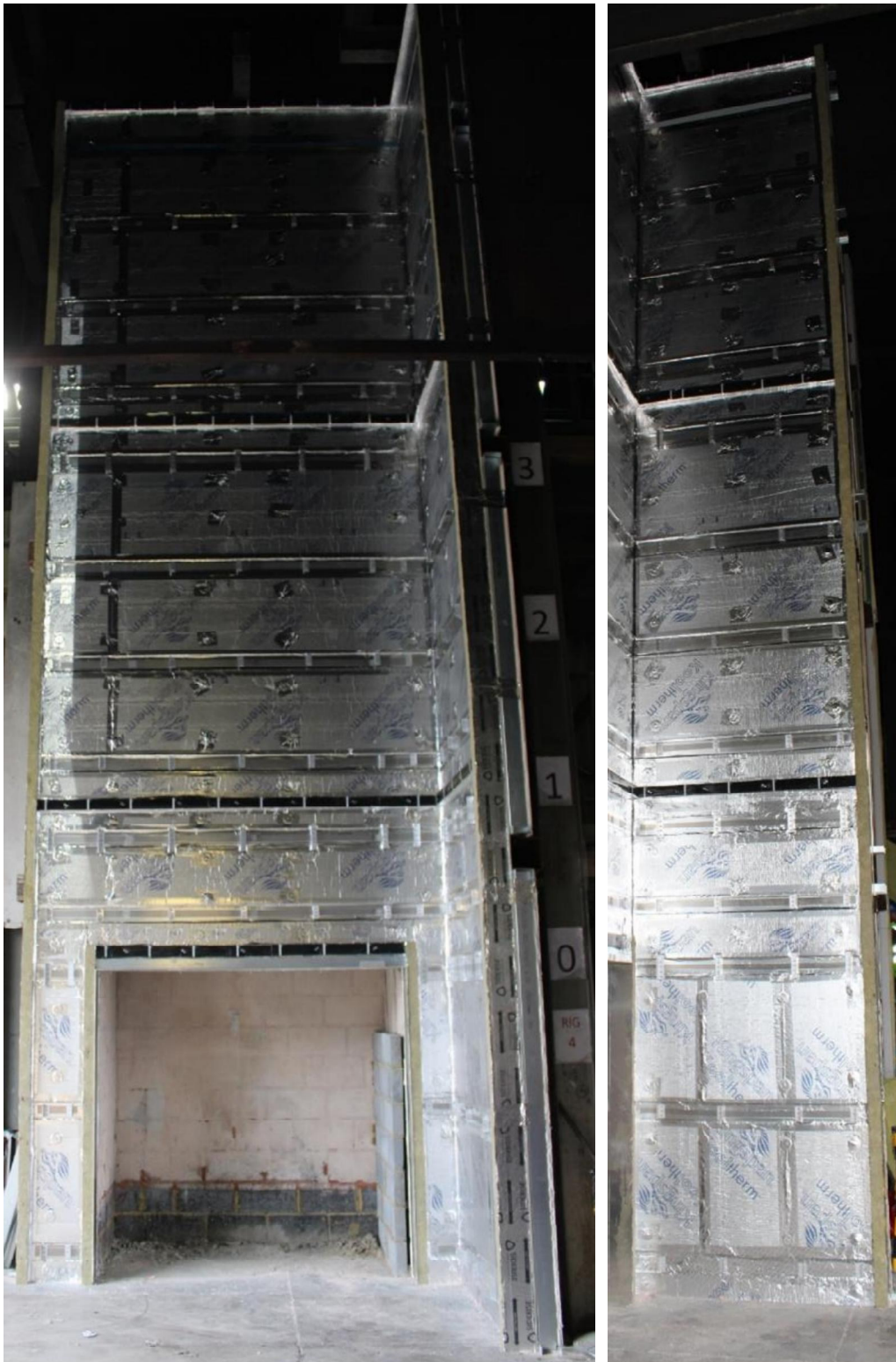
Figure 15. Installation of brackets.
