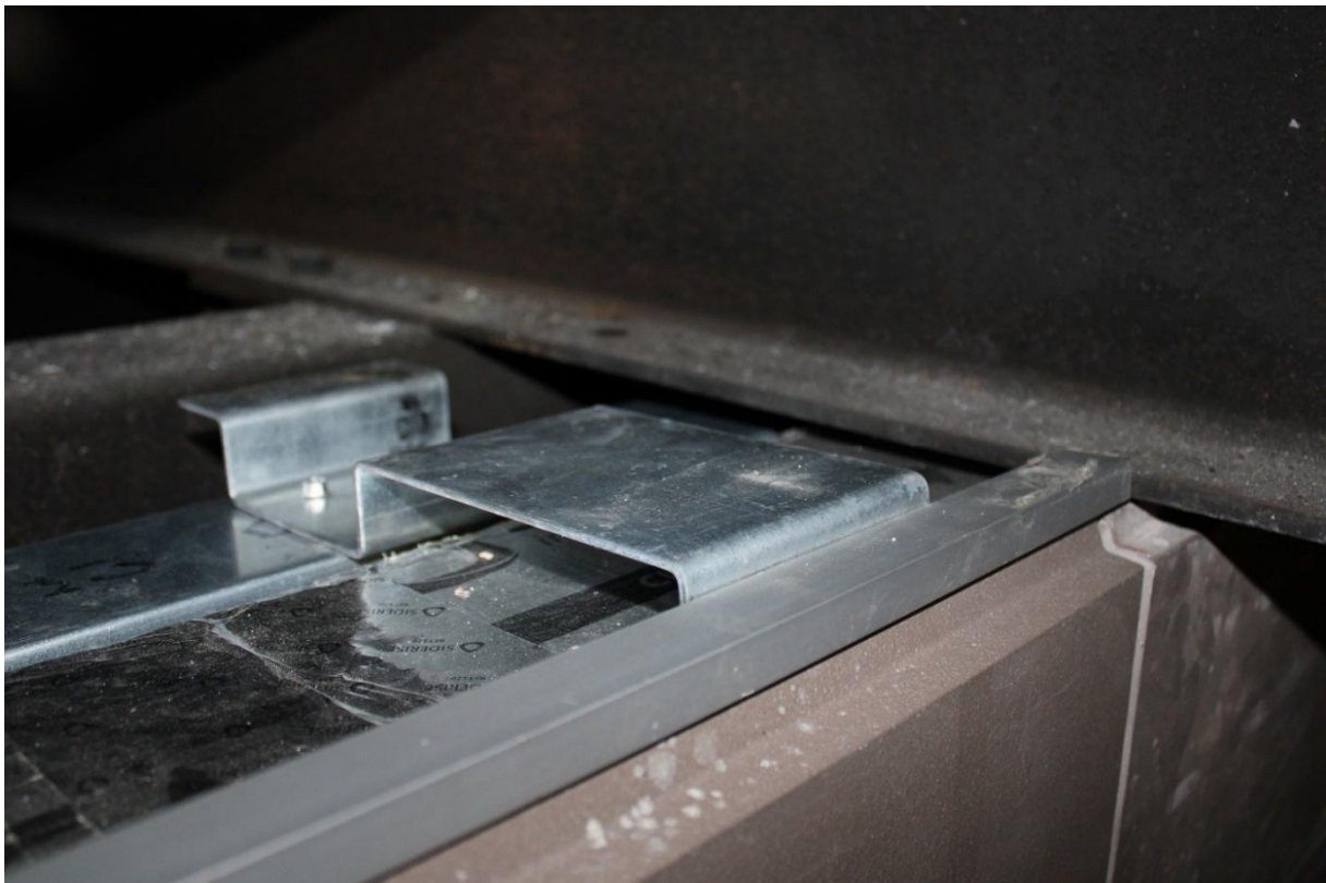
Figure 33. Top of system detail - profiled bracket and continuous top clip.
