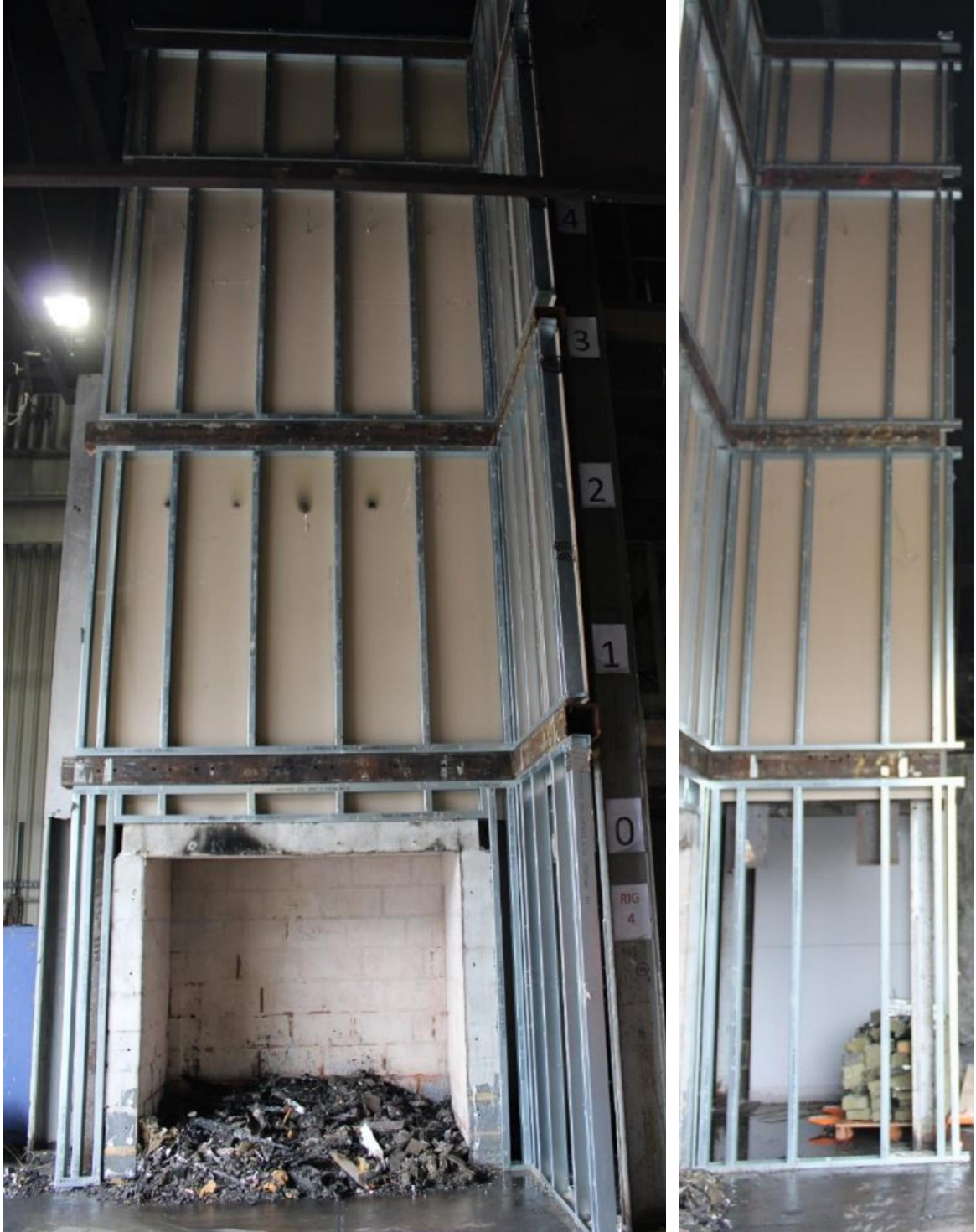
Figure 63. Full-height photograph of the steel framing system and plasterboard (exposed face).
