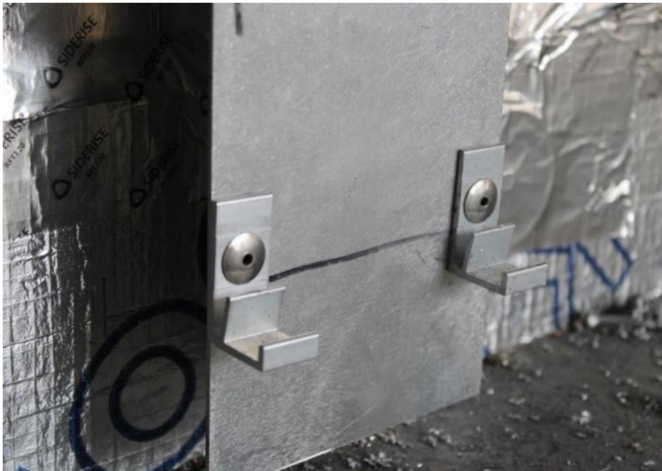
Figure 23. Base tile clip fixed to rails
