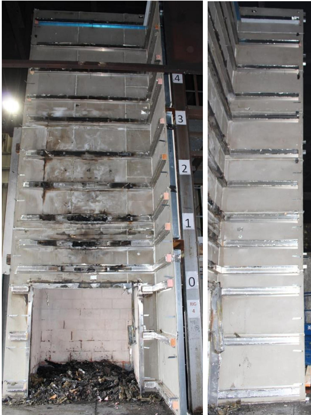
Figure 60. Full-height photograph following removal of cavity barriers.
