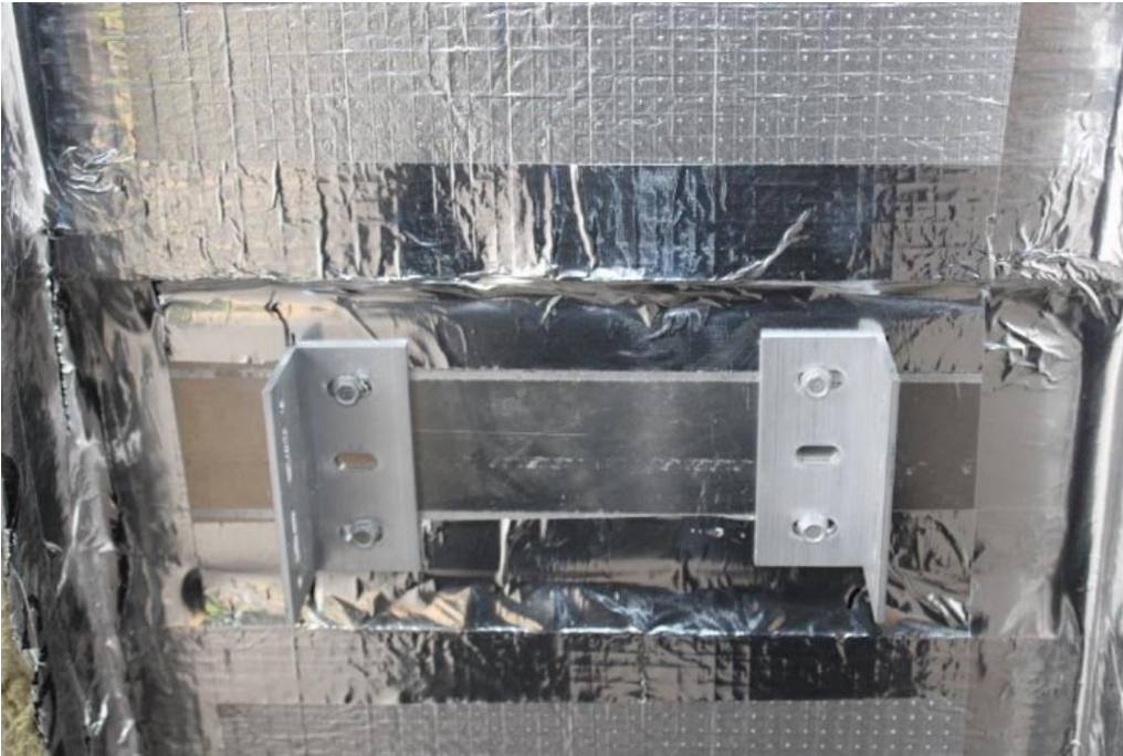
Figure 16. Single bracket.
