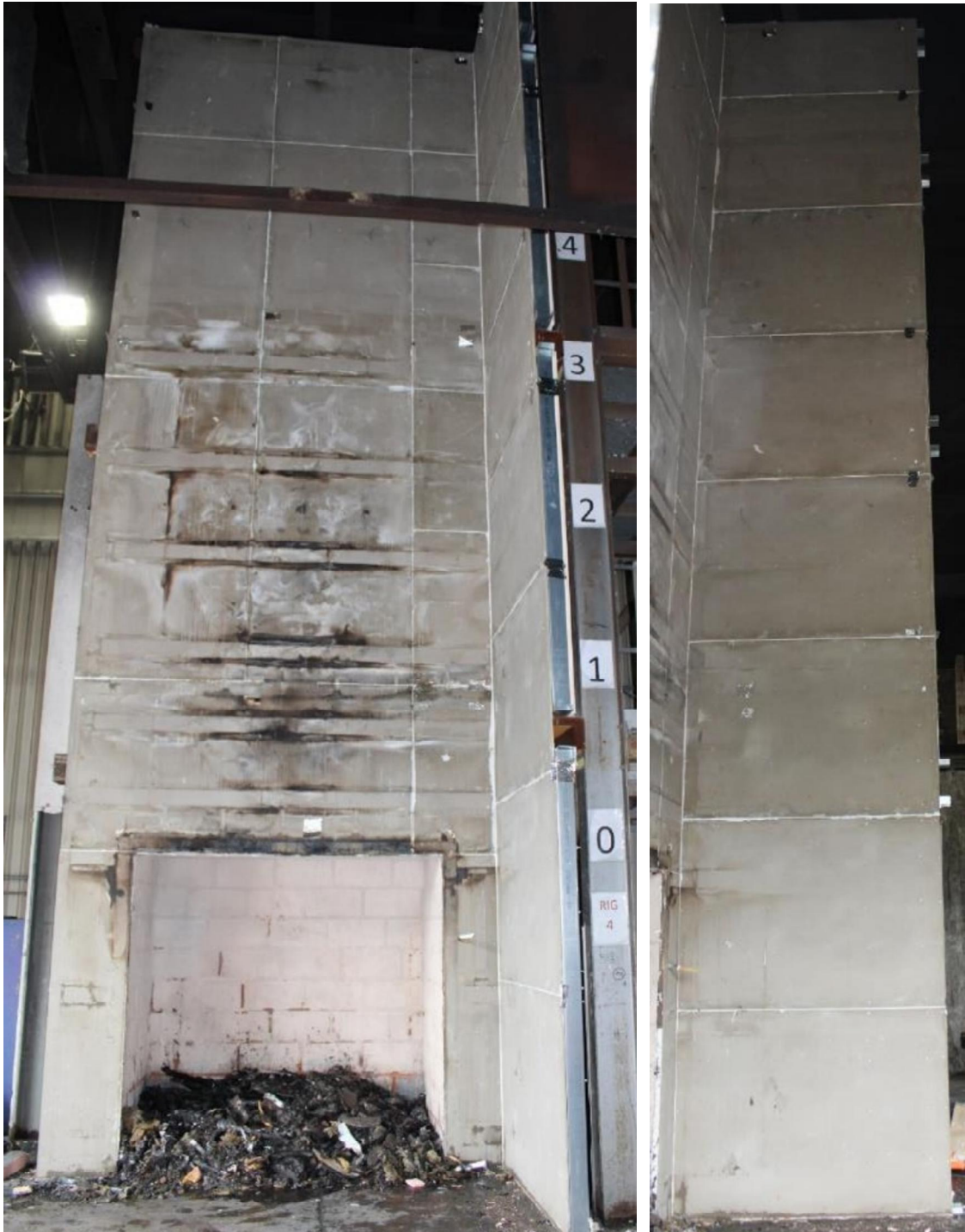
Figure 62. Full-height photograph following removal of the top-hat channels.
