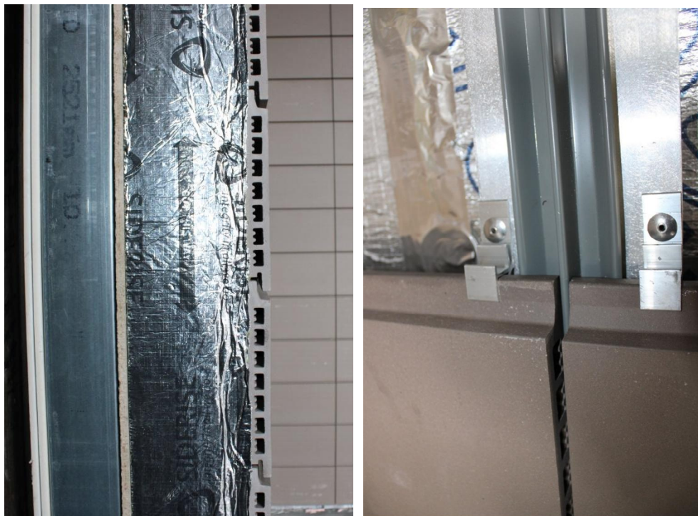
Figure 29. Installation of tiles.
