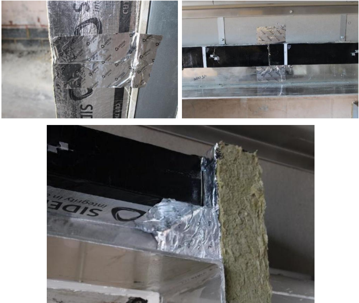
Figure 12. Horizontal and vertical cavity barrier joints.
