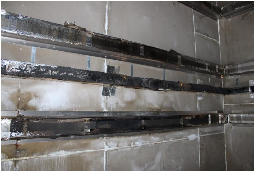
Figure 58. Photograph of the 2 nd full width horizontal cavity barrier.
