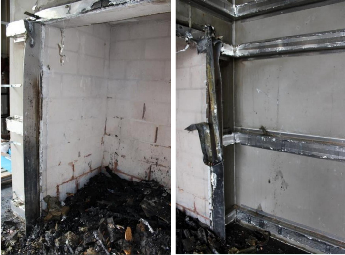
Figure 61. Photograph of combustion chamber surround flashing.
