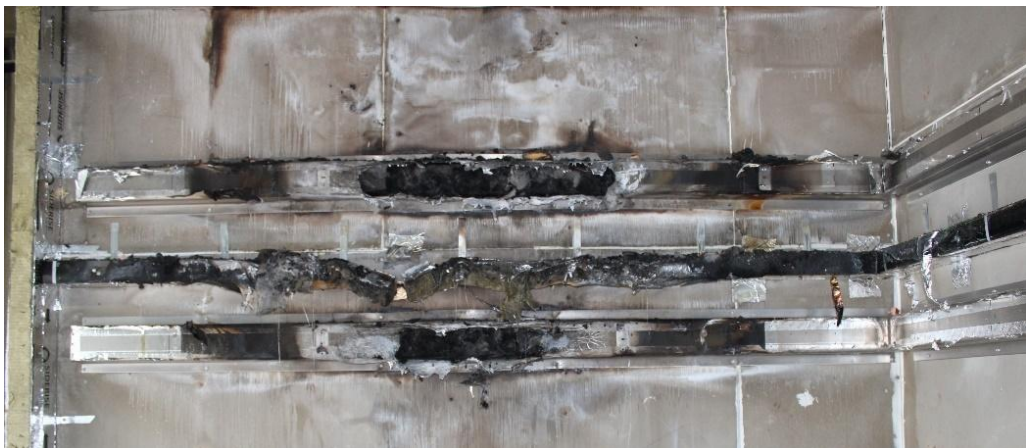
Figure 57. Photograph of the 1 st full width horizontal cavity barrier.
