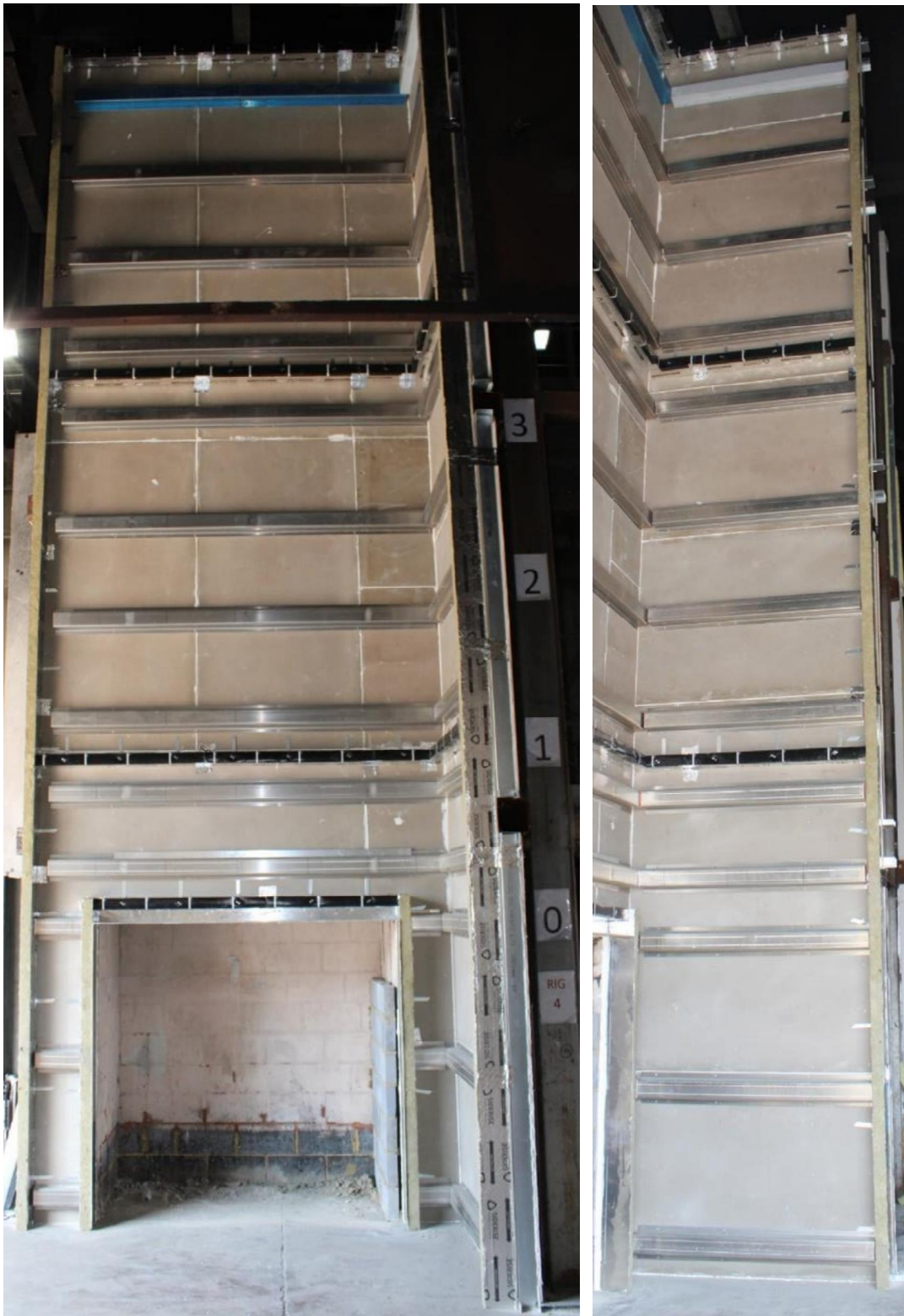
Figure 11. Installation of horizontal and vertical cavity barriers.
