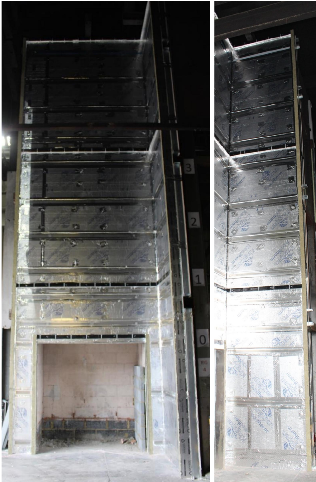
Figure 13. Installation of insulation.
