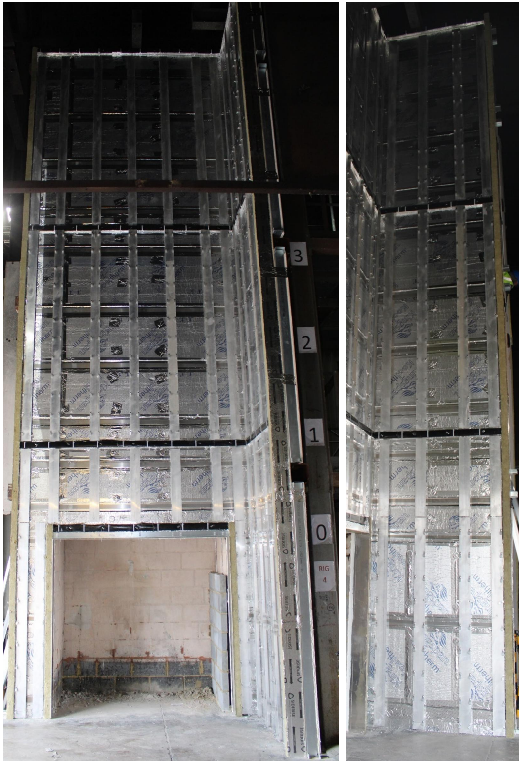
Figure 18. Installation of 'T'-shaped rails.
