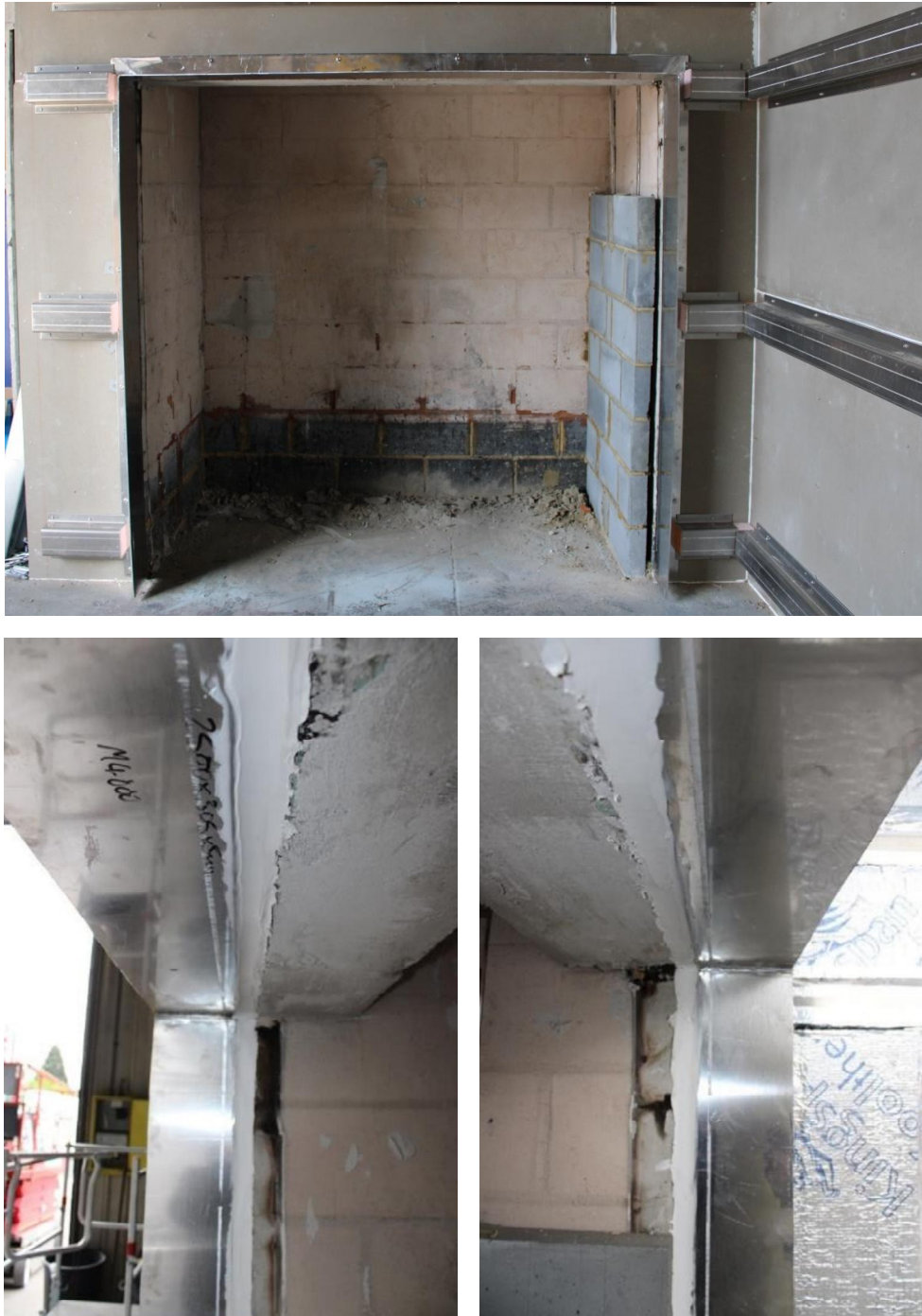
Figure 10. Installation of combustion chamber flashing.
