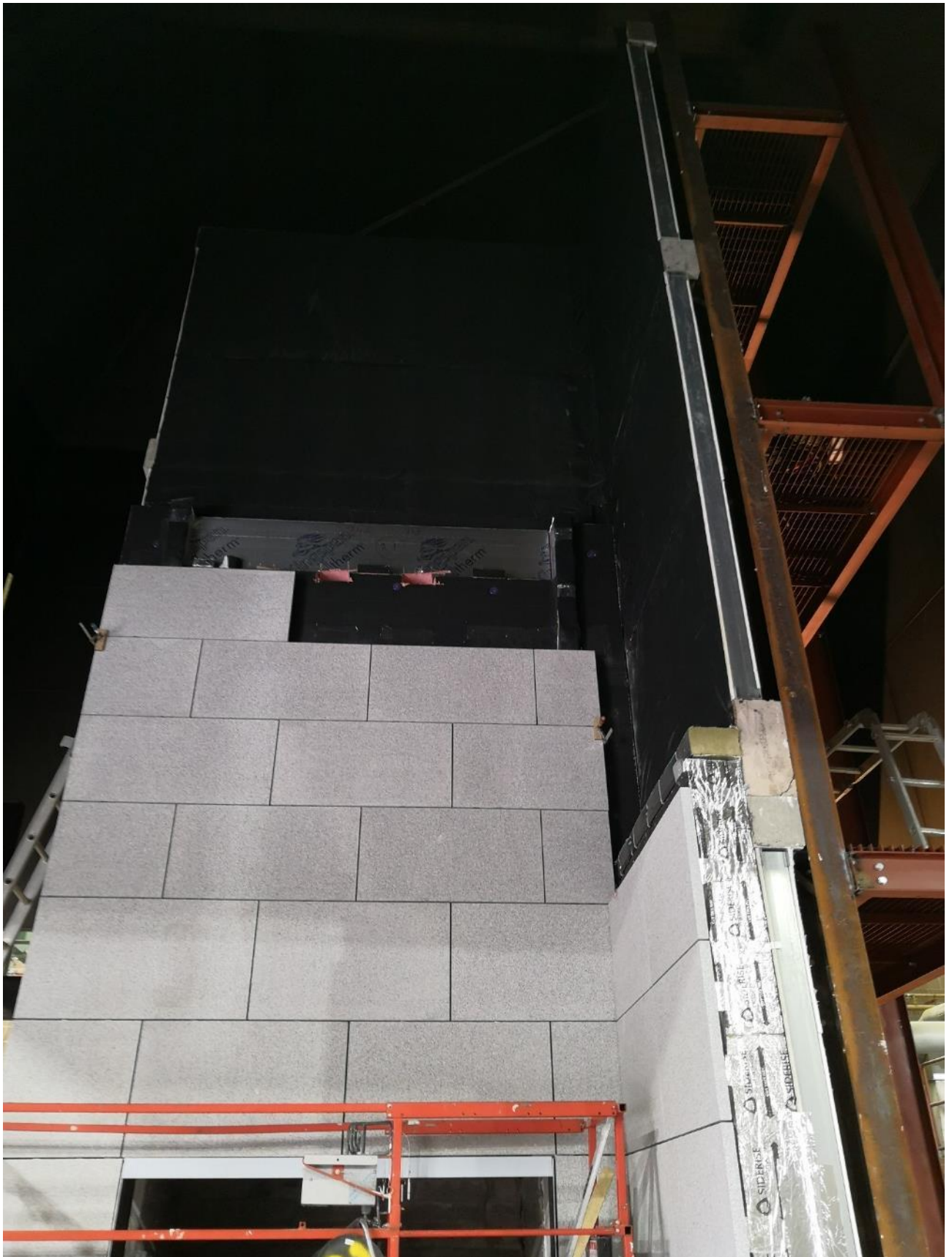
Figure 4.7. Installation of stone cladding panels during construction.
