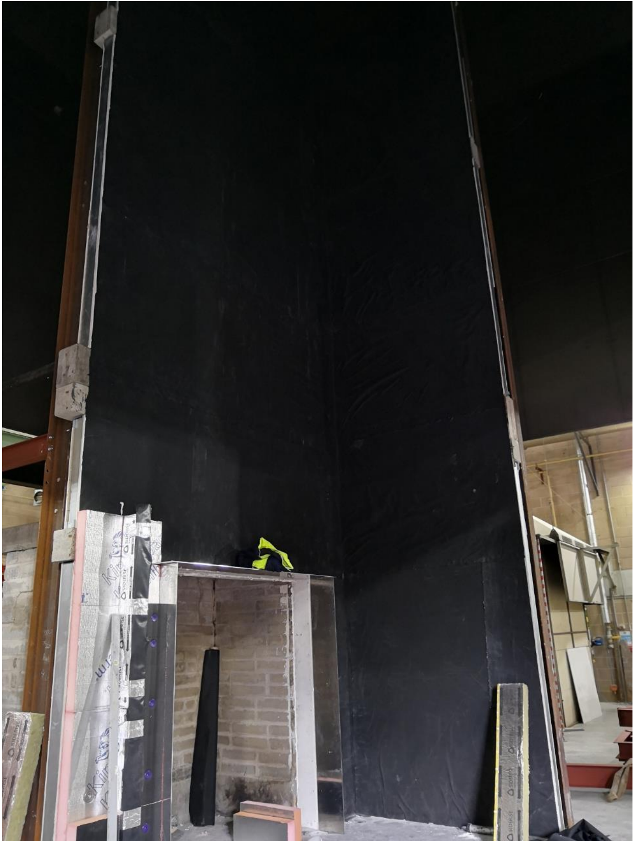
Figure 4.5. Installation of waterproof membrane completed during construction. Aluminum pod-frame also shown. Start of insulation and vertical fire stop barriers installation.
