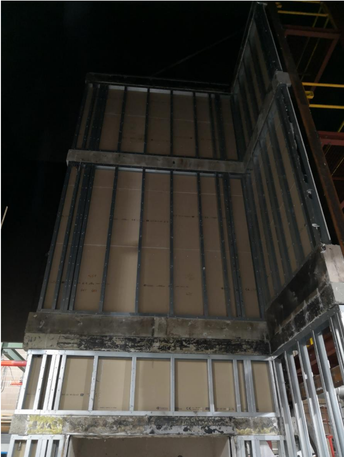
Figure 4.25. Post-examination damage. Photo of the system showing the plasterboard layer and SFS Kingframe after the test.
