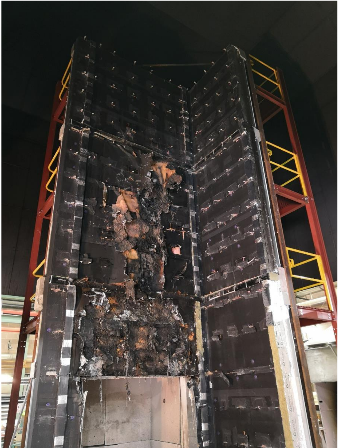
Figure 4.16. Post-examination damage. Insulation mainly charred and burnt above the combustion chamber on the main face; intact on the wing face. Vertical fire stop barriers in-place with some damage on the one located right of the chamber.
