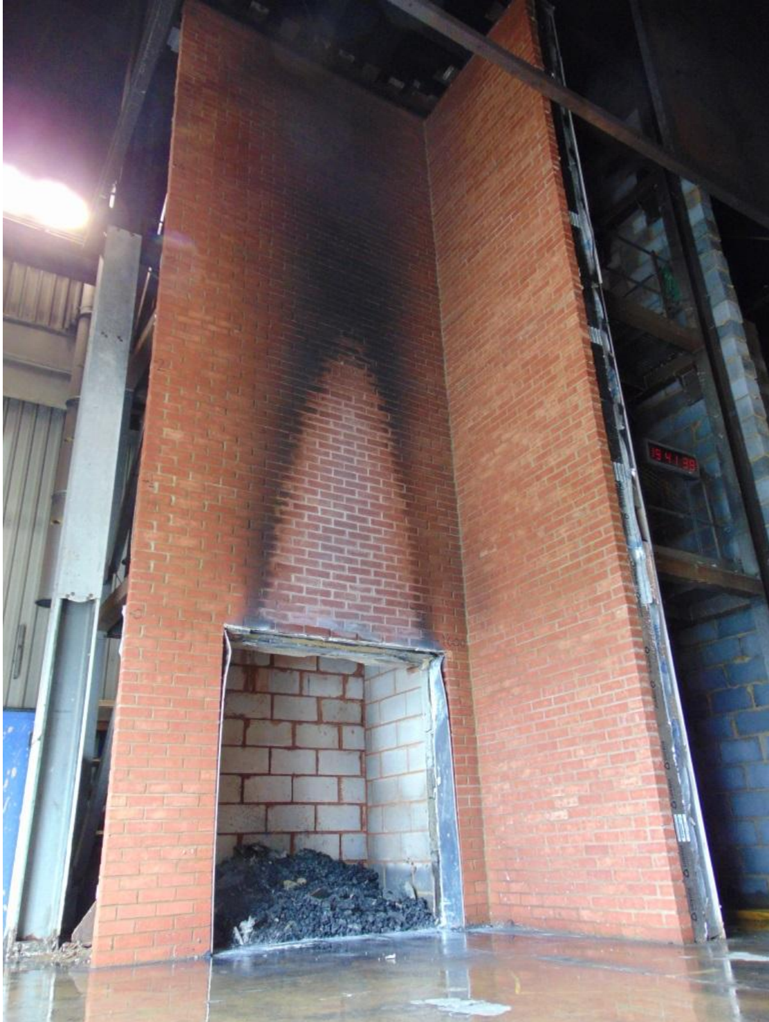
Figure 21. Full-height photograph of cladding system after test.
