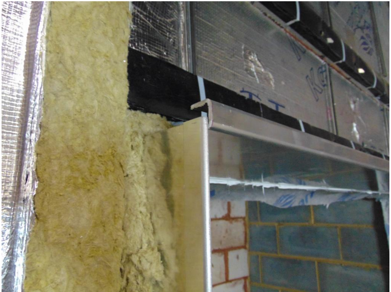
Figure 7. Combustion chamber surround flashing.
