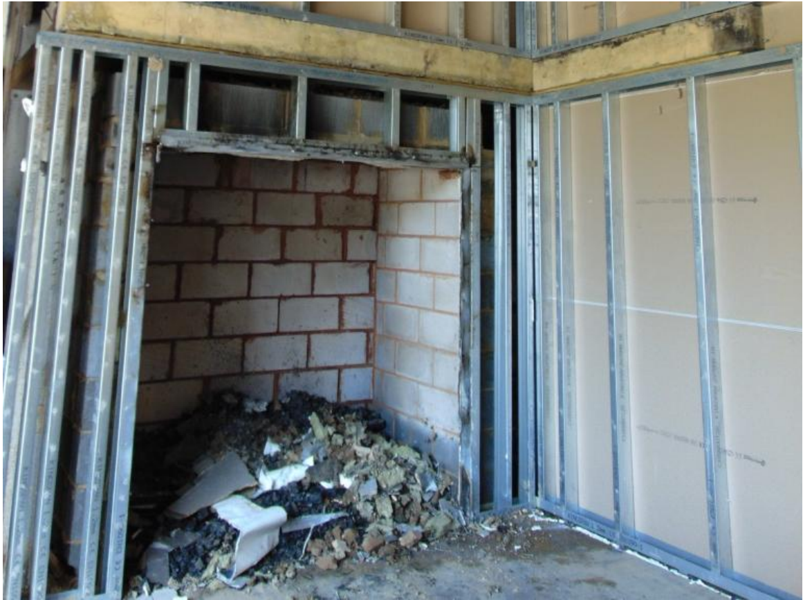
Figure 32. Lightweight steel framework partition from ground to first row floor slabs.
