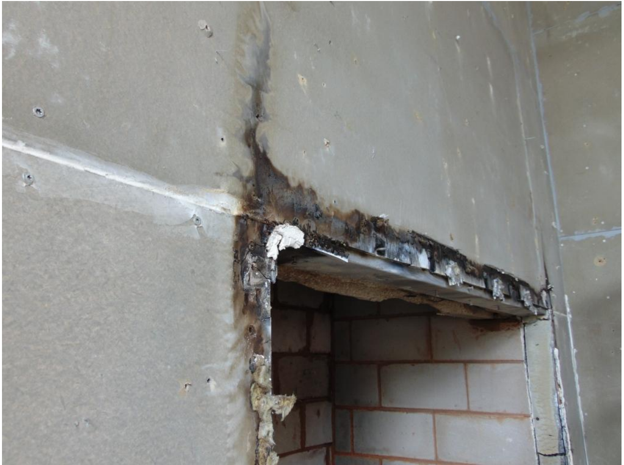
Figure 30. Cement particle board immediately surrounding combustion chamber.
