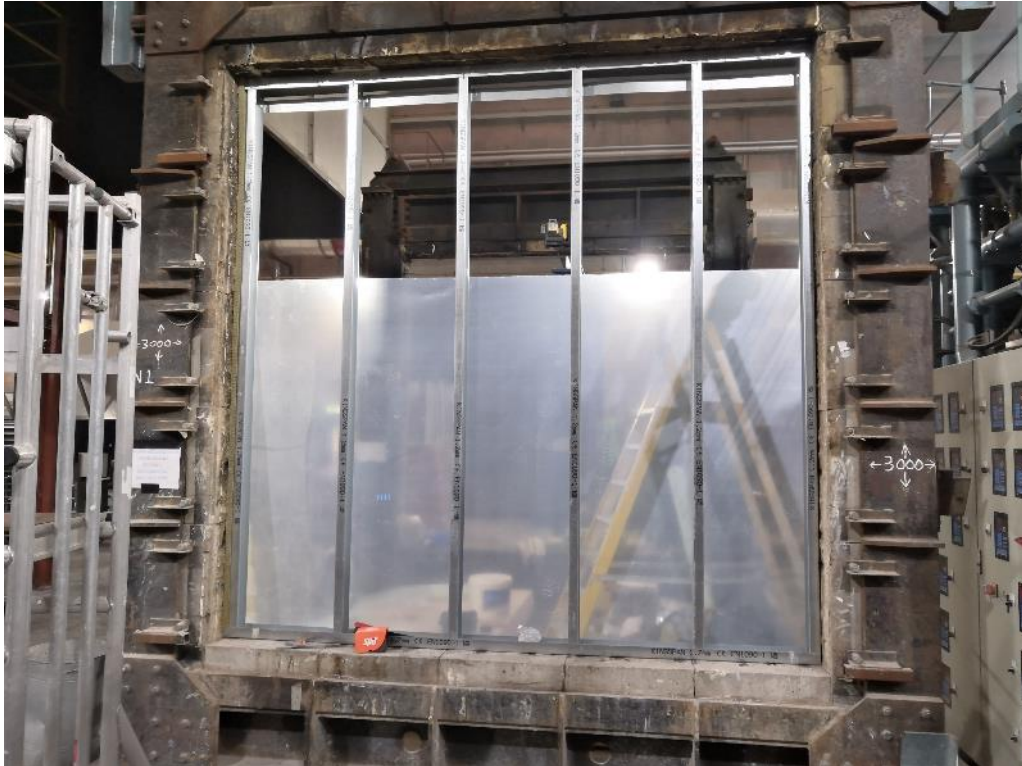
Photograph 1 – Overall view of the sample frame during construction (viewed from the unexposed side). Note the layout of the frame and the installation of part of the VCL membrane – free edge on the left-hand side
