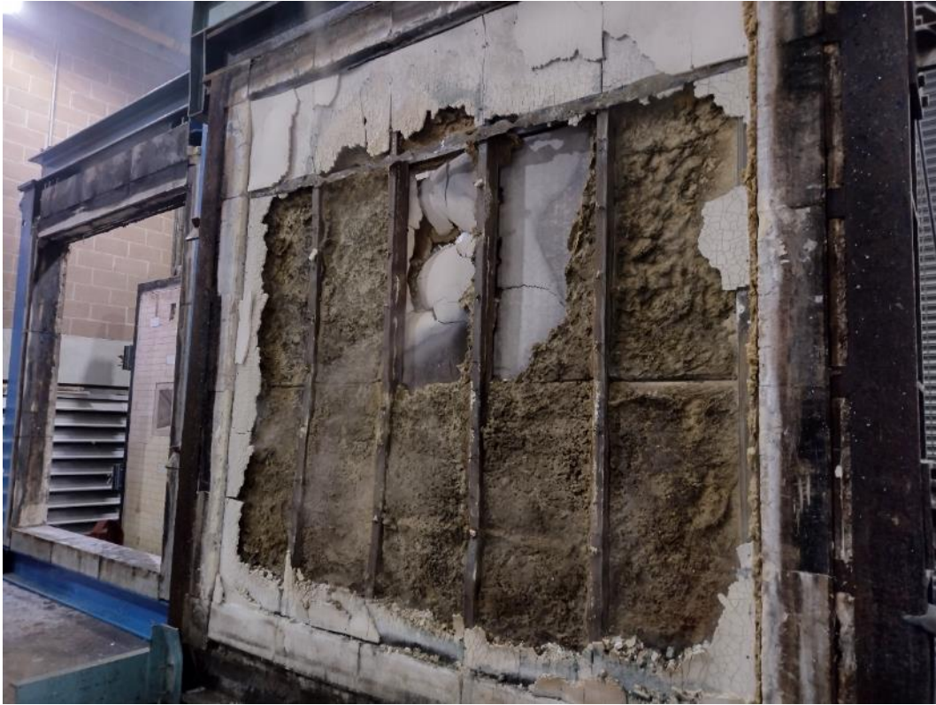
Photograph 15 – Overall view of the exposed side of the sample after cooldown and removal from the furnace.
