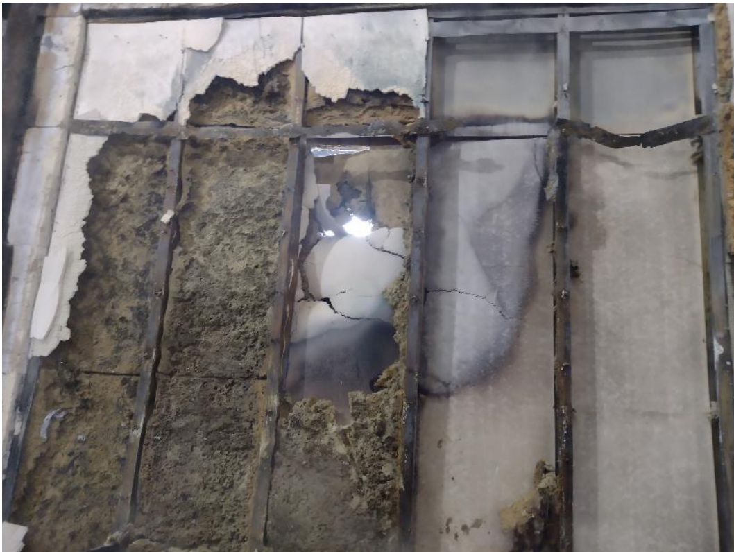
Photograph 16 – Detail of the exposed side of the sample after cooldown and removal from the furnace. Note the discolouration on the sheathing boards, visible after removal of the insulation.
