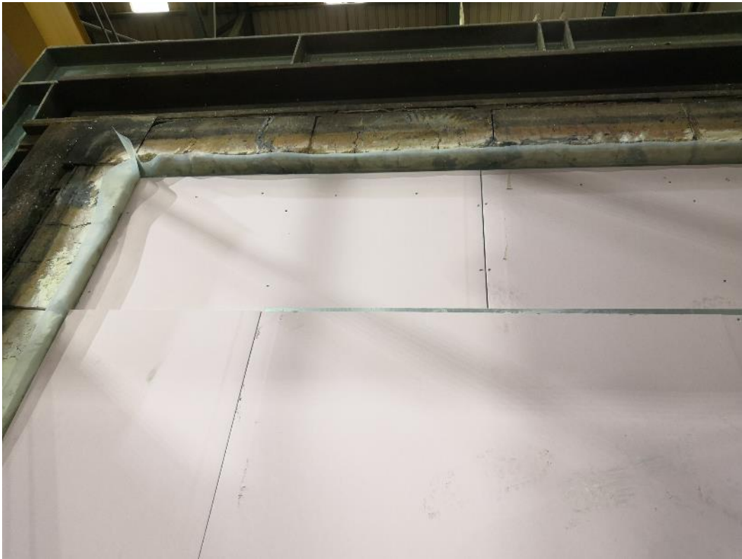
Photograph 3 – Detail of the exposed side of the sample during construction. Note the location of the fixing strap and staggered layout of the boards between layers.
