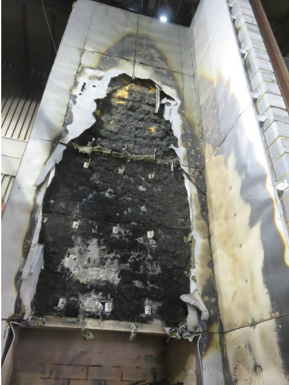
Figure 14. Full-height photograph immediately after test.
