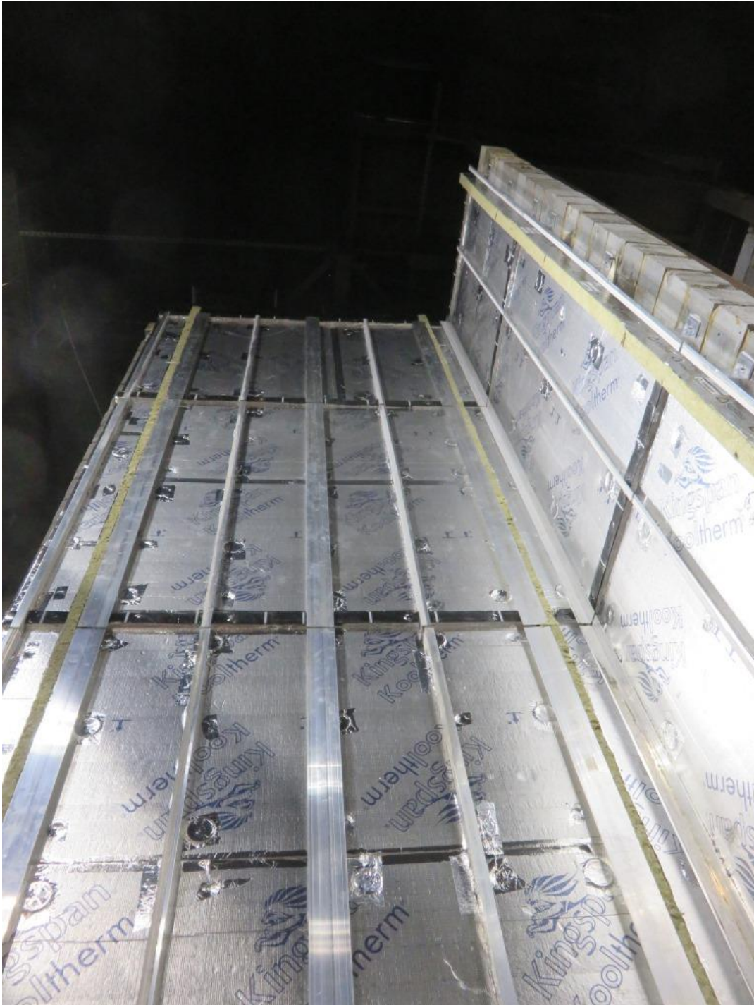
Figure 6. Completed installation of Allface System F1.10 aluminium rail substructure.
