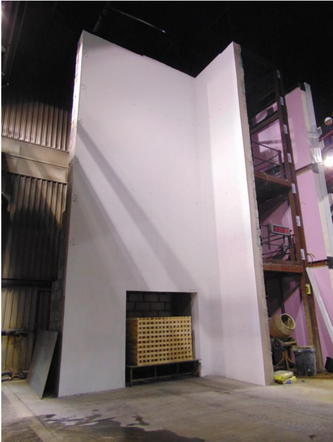
Figure 1. Cladding system prior to test.
