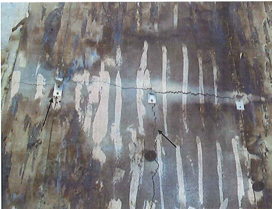
DLP C2753J/0018 Brackets and cement particle board
