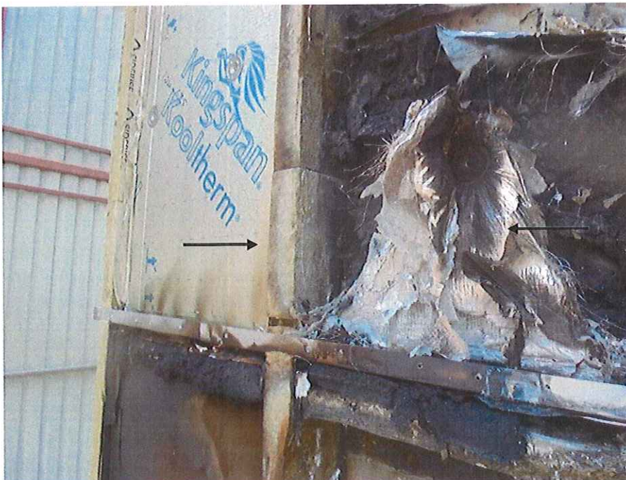
DLP C2753J/0016 Vertical cavity barrier, insulation and railings on main wall
