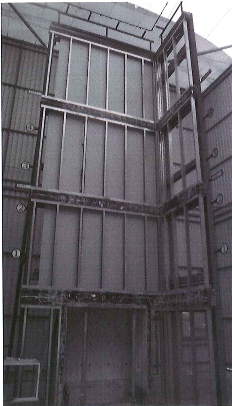
DLP C2753J/2383 100mm Kingframe SFS and plaster board
