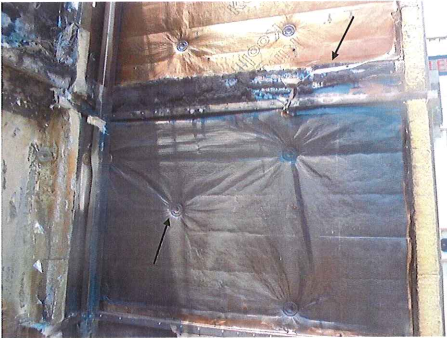
DLP C2753J/0017 Cavity barrier, insulation and railings on wing wall
