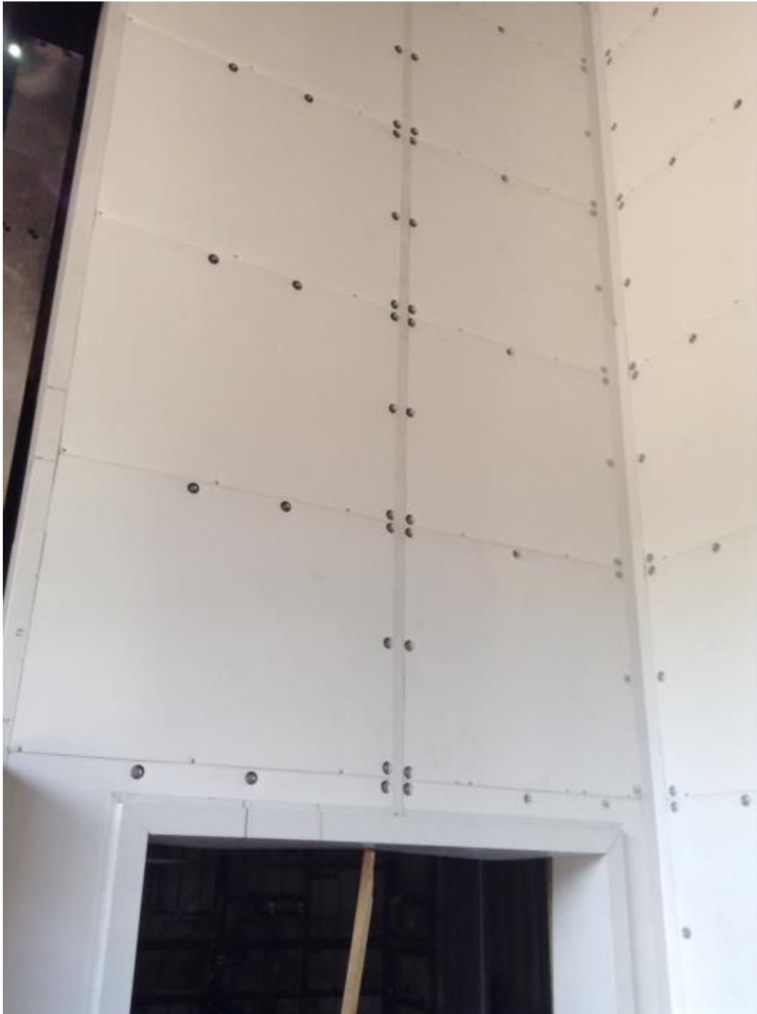
Figure 1. The system during construction.
